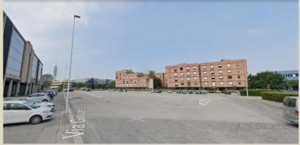
The square has an area of approximately 6800 square metres and was entirely paved with bituminous conglomerate and therefore completely impermeable.
